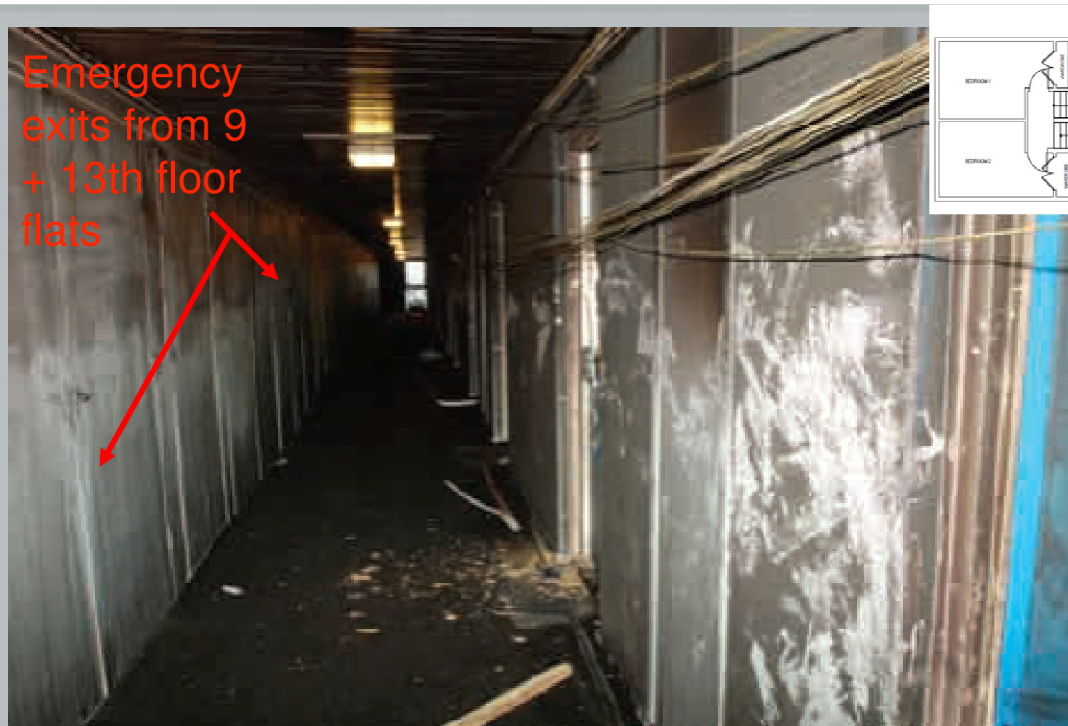
Fig 30: Post incident photograph showing conditions on the eleventh floor after the escape door from Flat 72 was left open. Note the displaced cables. (Source: Hampshire Constabulary)
