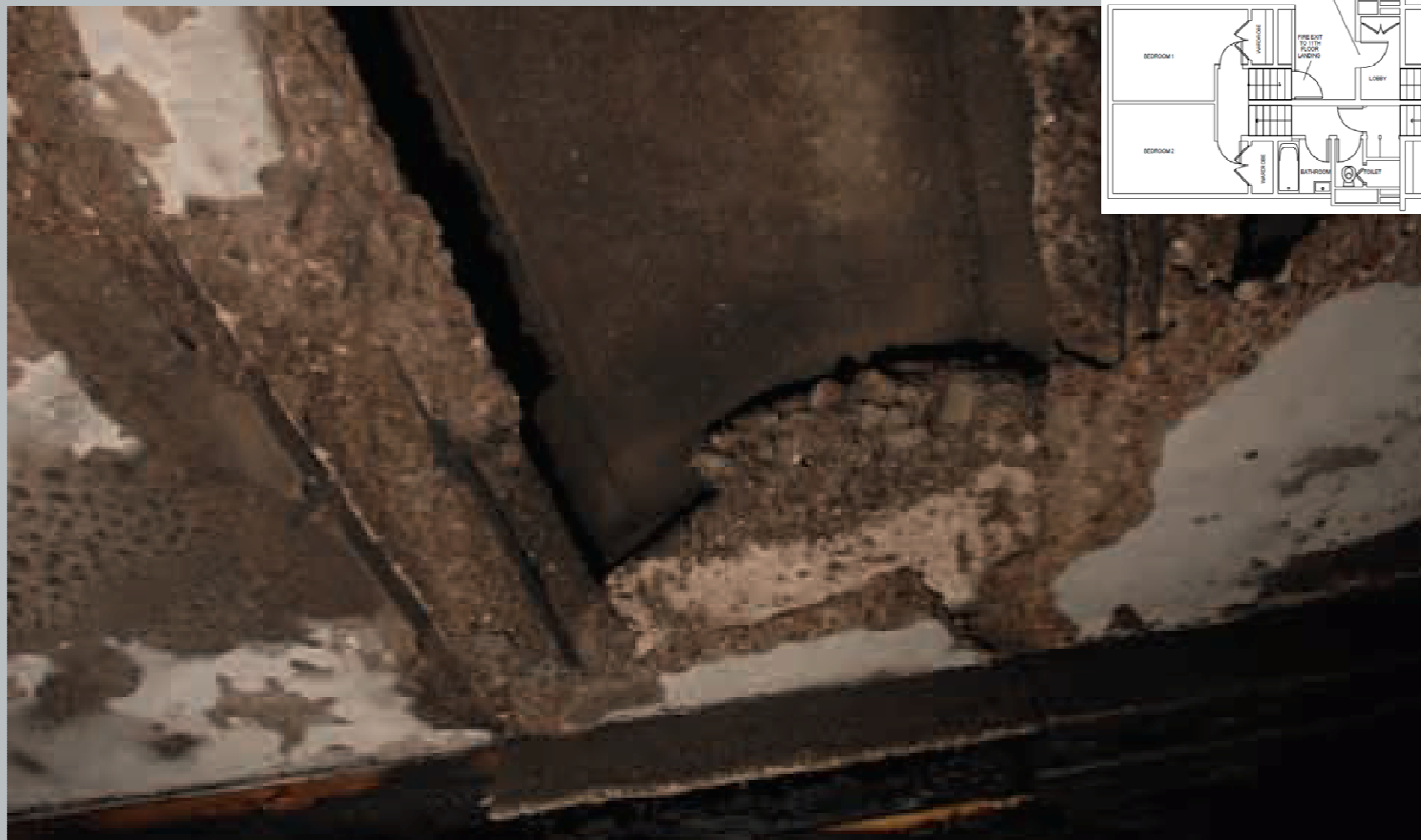
Post incident photograph of kitchen ceiling showing the fire damage to the concrete beams (Source: Hampshire Constabulary)
